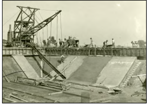
Construction of the Coal Pit.
